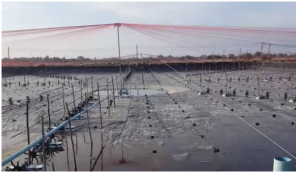
Fig.1 Grow-out shrimp pond with plastic sheet liner 100% and sump (8-m diameter, 2.5-m deep) Source: Thai Shrimp News (2017)
